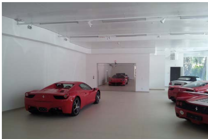
TRAFFICO® Garage Zenith SA, Sion, Switzerland
