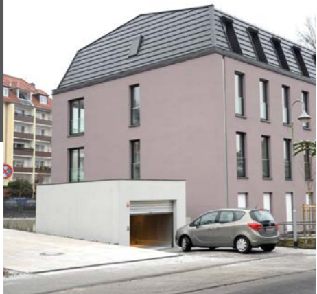
PEGASOS®, apartment building, Königstein, Germany
