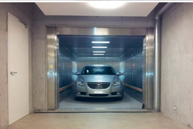
TRAFFICO® Parking, Zürich, Switzerland
